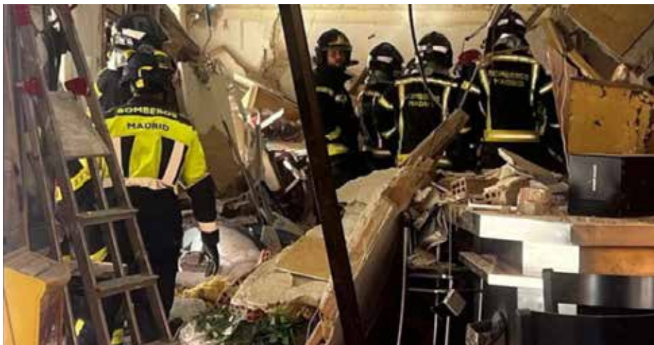
Foto von Madrid Fire Services
